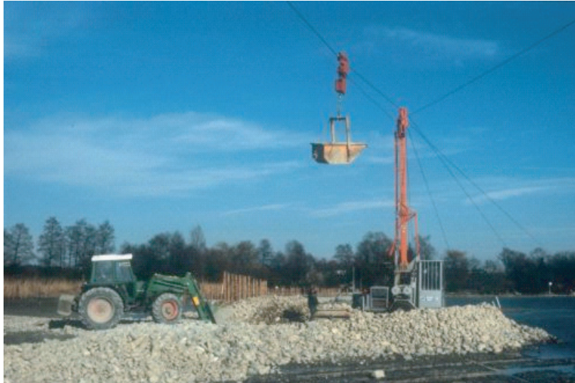
Fig. 5. Lakeshore rehabilitation works during low water period in February. Here, an eroded beach is filled up with a basement of boulders to give a break wave construction.
