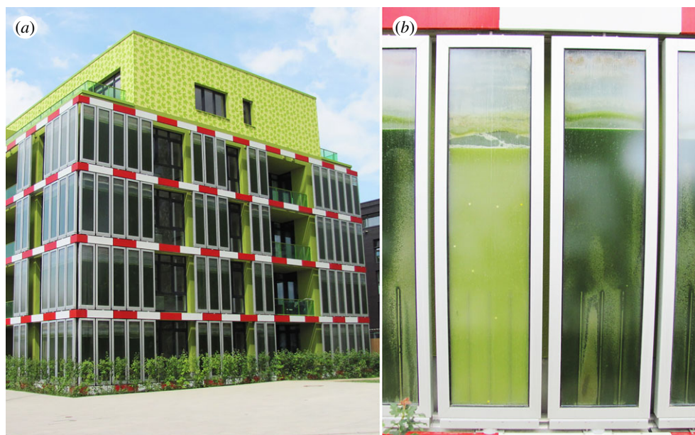
Figure 4. The BIQ Algae House [200] with algae façade panels by Elsayed et al. [201] that cultivate biomass for energy production. Left and right images both used with license. (Left image, titled 'IBA Hamburg BIQ (2).nnw.jpg', and right image, titled 'IBA Hamburg BIQ Fassadenteil mit Mikroalgen.nnw.jpg', are both retrieved from Wikimedia Commons, both from username NordNordWest. Both images used with Creative Commons license CC BY-SA 3.0. Image copyright holder for both images chose and approved the licenses at upload.) (Online version in colour.)
