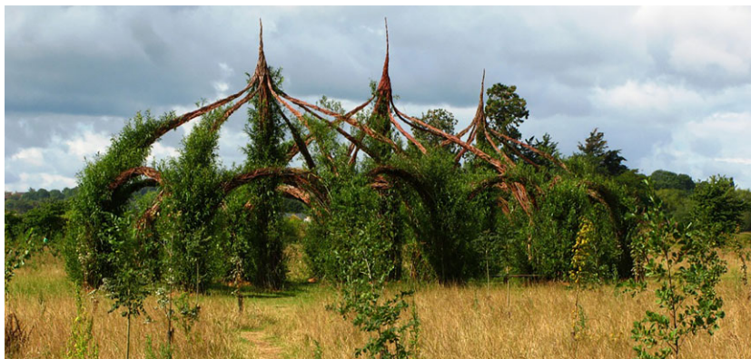
Figure 6. The Longrun Meadow Willow Cathedral , 15 an example living willow structure, built by permanently constraining the willow in large bundles; image used with license. (Image retrieved from Wikimedia Commons, from username Geof Sheppard. Used with Creative Commons license CC BY-SA 3.0. Image copyright holder chose and approved the license at upload.) (Online version in colour.)
