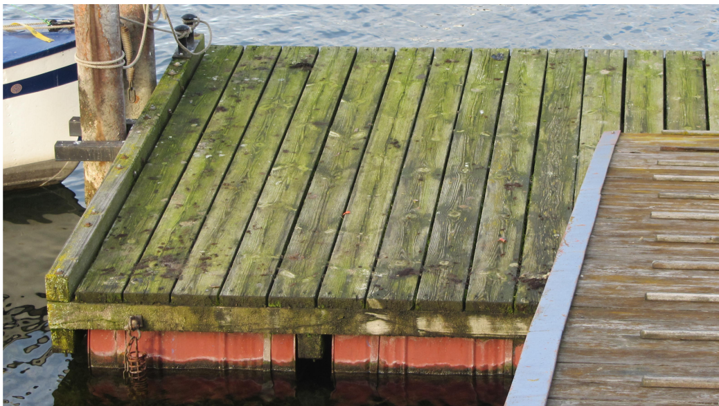
Figure 1.1: Formation of photoautotrophic biofilms on various human made surfaces. (The picture was taken in January 2014 by M. Windler).
